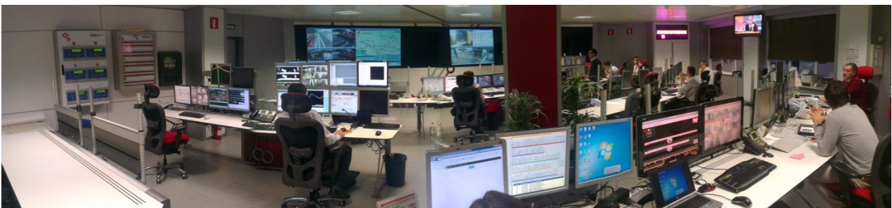
Figure 3. Security & Civil Protection Centre (source TMB)
